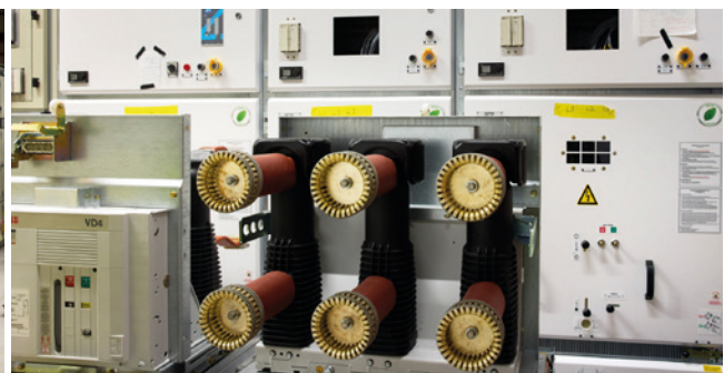
Upgrading with medium voltage switchgear from Harju Elektek at SSAB in Luleå. Switchgear from Aktif, breaker from ABB.
