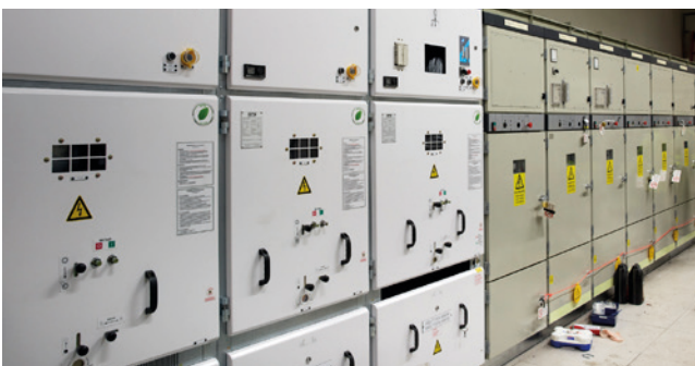
Upgrading with medium voltage switchgear from Harju Elektek at SSAB in Luleå. Switchgear from Aktif, breaker from ABB.
