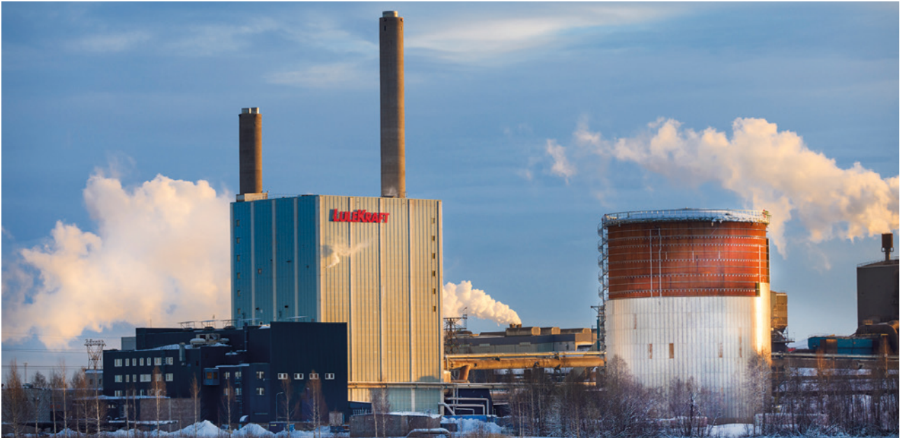
District heating is produced in the Lulekraft CHP plant.
